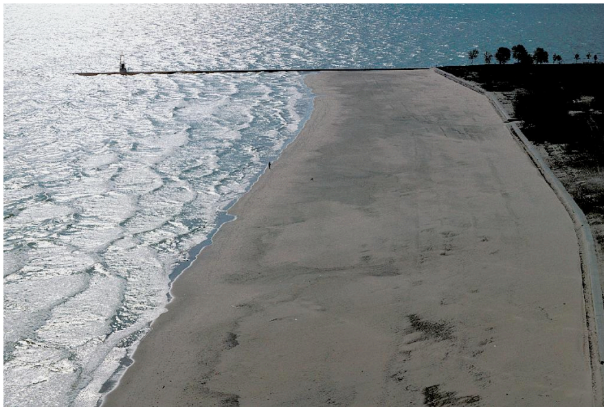
Figure 7. Jetty at Chicago, Illinois, along the Lake Michigan coast. Note the accretion (or beach growth) in the foreground of the picture, and the absence of a beach beyond the jetty. As this photo illustrates, jetties interrupt the natural flow of longshore sediment transport. Image Source: Earth Science World Image Bank http://www.earthscienceworld.org/images
